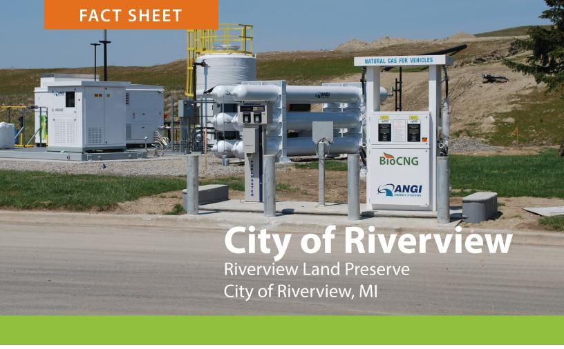
BioCNG, LLC, is part of a team that assisted with the development of a BioCNG™ alternative vehicle fuel system at the City of Riverview's Riverview Land Preserve (RLP). BioCNG provided site design and permitting services, and furnished the biogas conditioning system, the compressed natural gas (CNG) fueling station, and the CNG storage tanks. BioCNG also performed system commissioning and startup.
